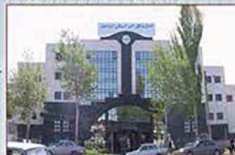
Central water supply office in Ardabil
