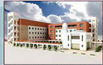
Supervision of Buildings Complex of Yazd
