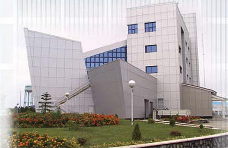
Inspection of ports and shipping administrative building of Gilan province
