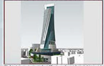
Elahieh commercial, office and residential complex
