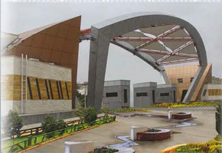
Gate way of Petro leum in Mahshahr port
