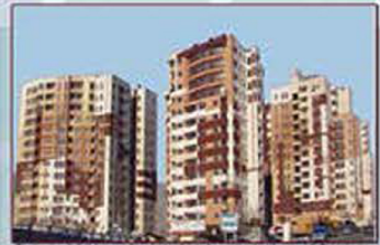
General inspection on implementation of Sarve complex high rise buildings (18 stories)
