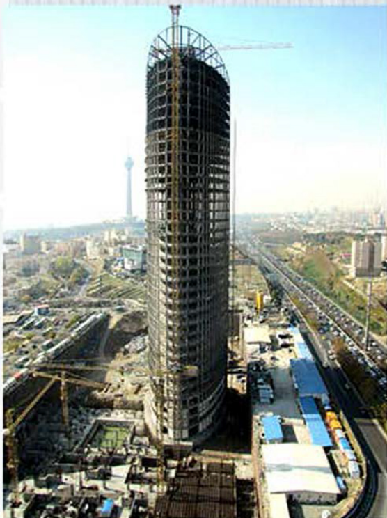
High supervision of construction of the company's telecommunication companies
